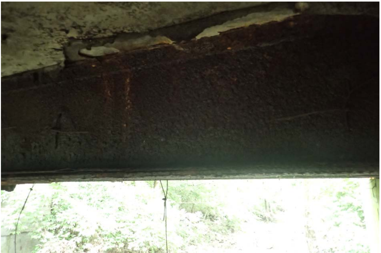
Beam 4 near the east abutment.
