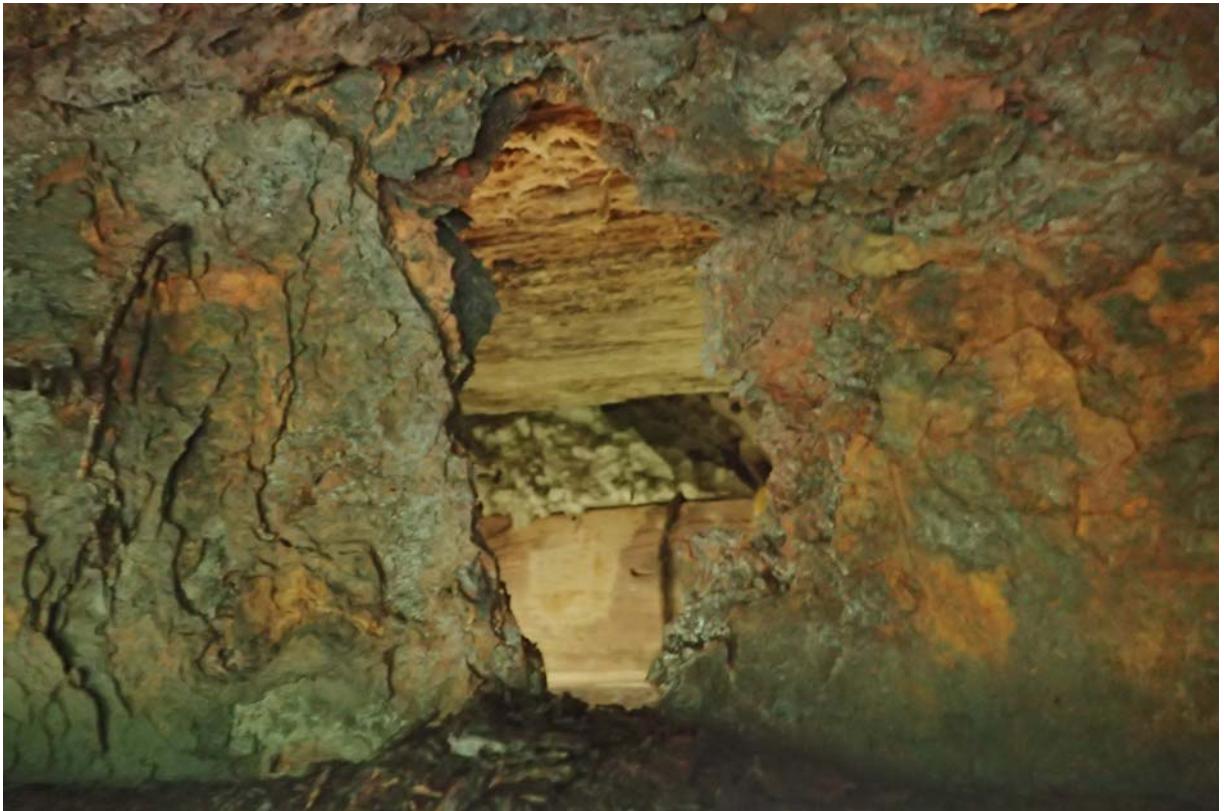
Full height rust through hole in the web of beam 4 from upstream near midspan.
