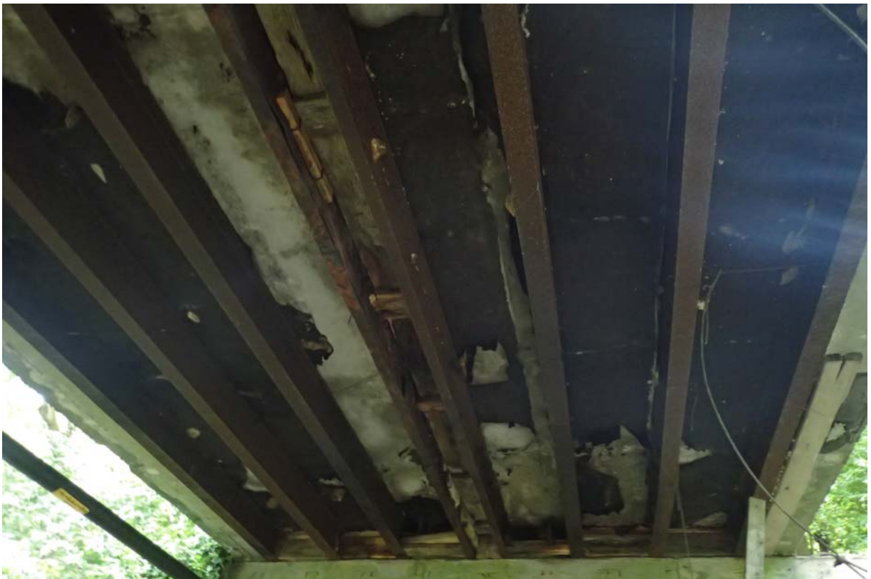
Beams and deck underside.
