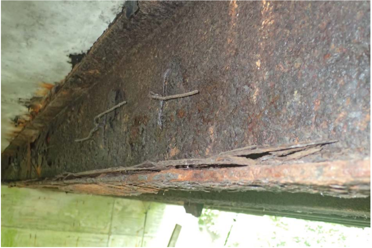
Sighting along beam 4 near the east abutment.
