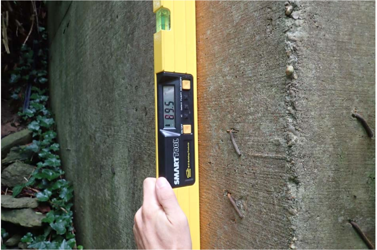
Smart level measurement on the downstream east wingwall.
