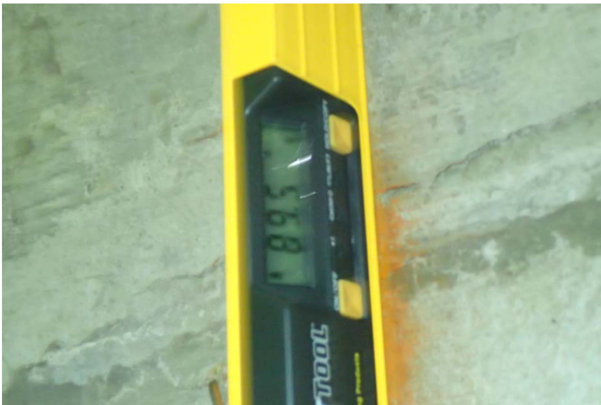
Smart level measurement on the downstream west wingwall.
