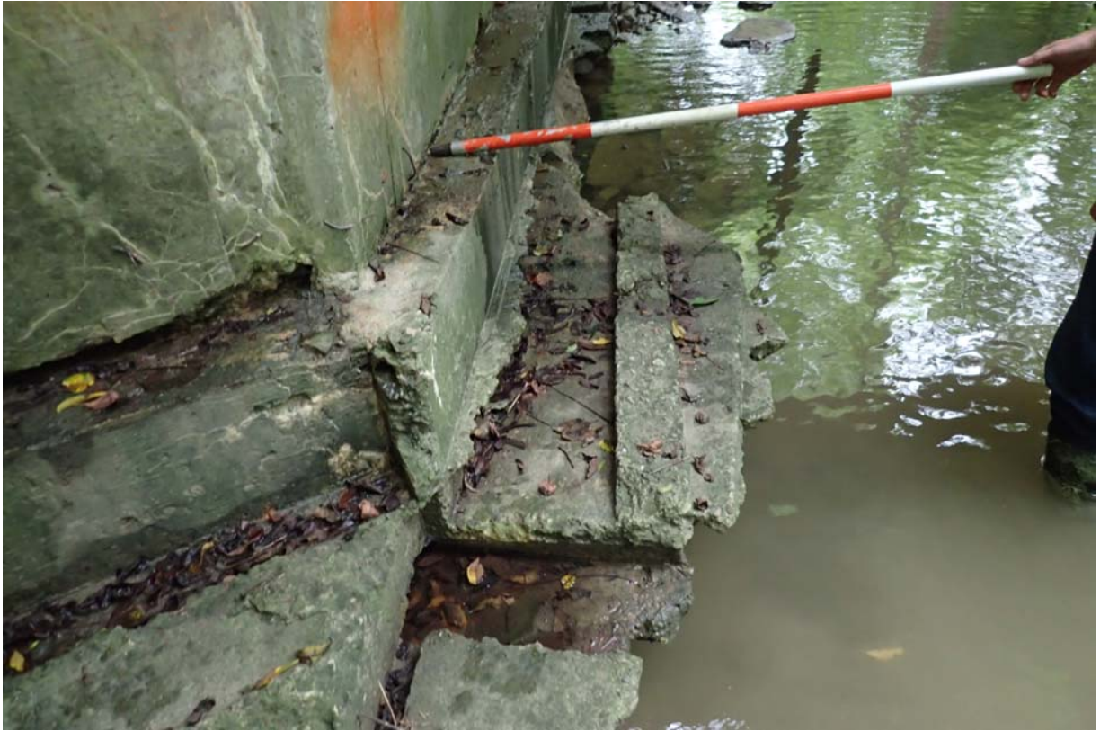
Approximate width of west abutments footing/apron.
