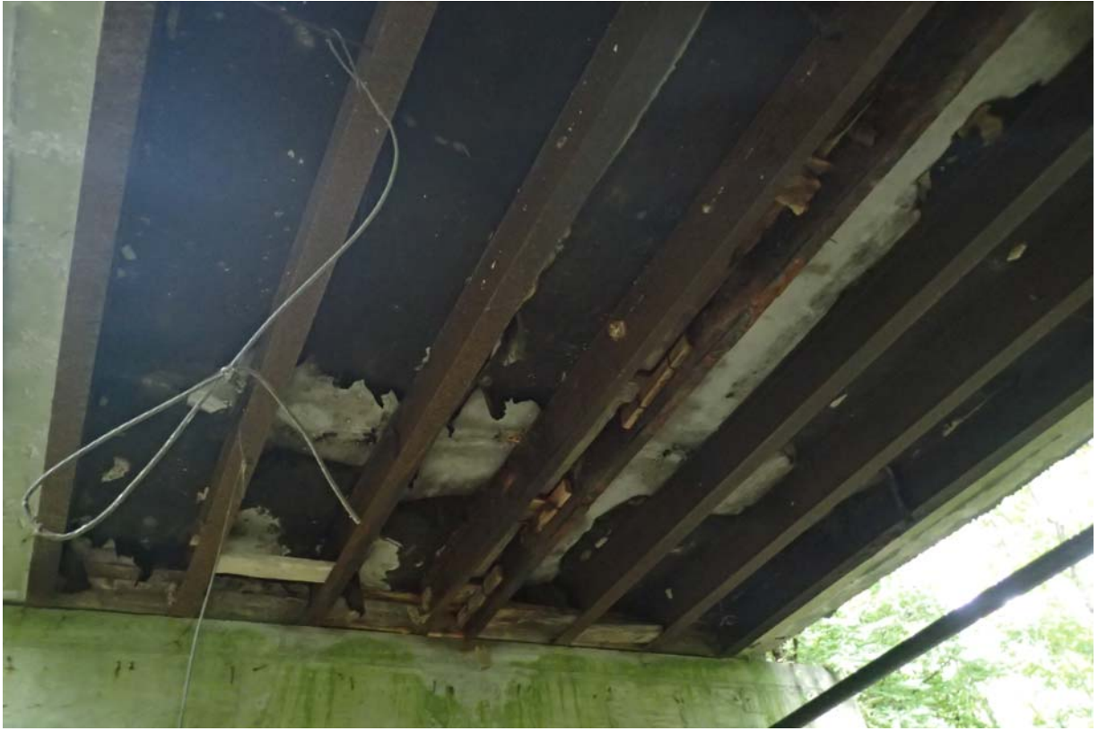
Beams and deck underside.
