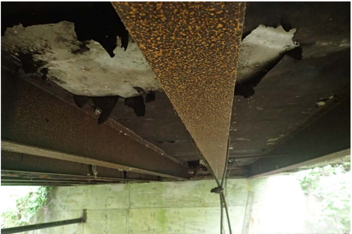
Sighting along beam 7 from upstream. Notice the bow in the downstream direction.
